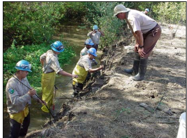
A CCC crew installing willow stakes and bundles to stabilize the stream bank at Chorro Flats.
