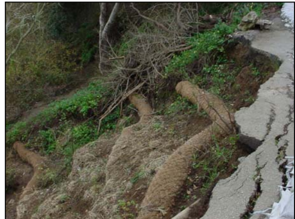
Chorro Creek Bank Stabilization – native plants and trees were planted between the bio-logs.
